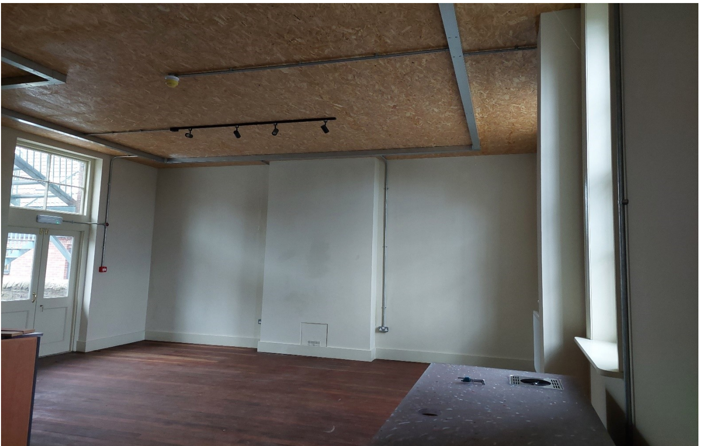
- Ground floor room –
