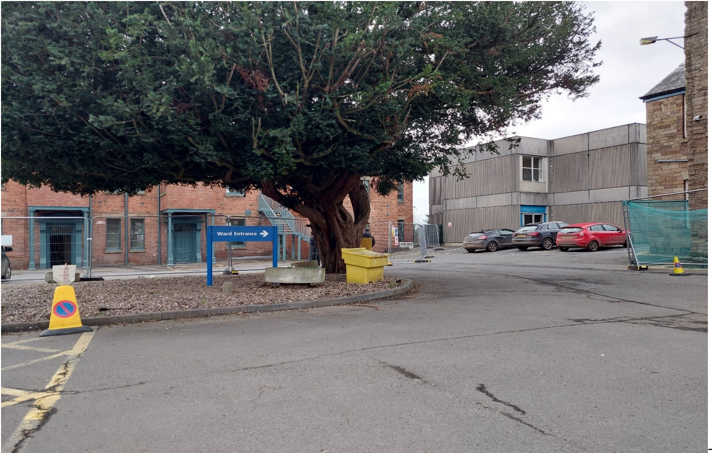
- Entrance to car park, detached building to right is part of Hospital –
