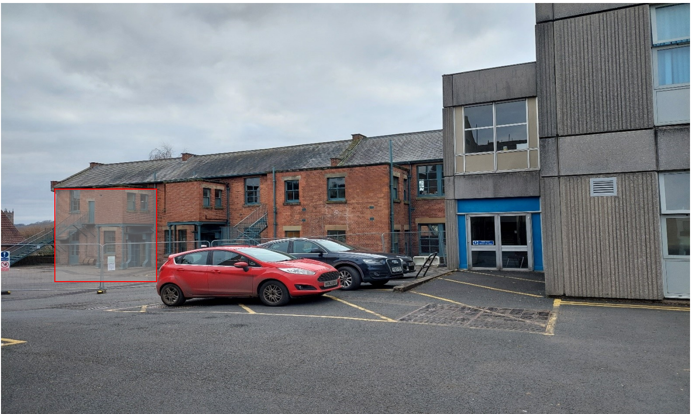
- View of premises, red online is part of premises applied for to be licensed, detached building to right is part of Hospital -
